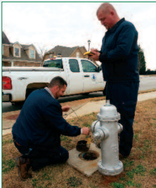
The HCWSA Leak Detection Program, through the work of its team members, has saved the Authority and its ratepayers approximately $933,000. (Above) The Authority's Gary May and Lee Mooney, employees on the leak detection team, check for leaks within the HCWSA system.
